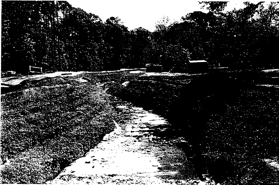
Figure 7. Three Months After Construction.
