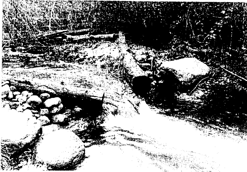
Figure 2. Timber Stepdown K-Structure (shown with weir logs).
